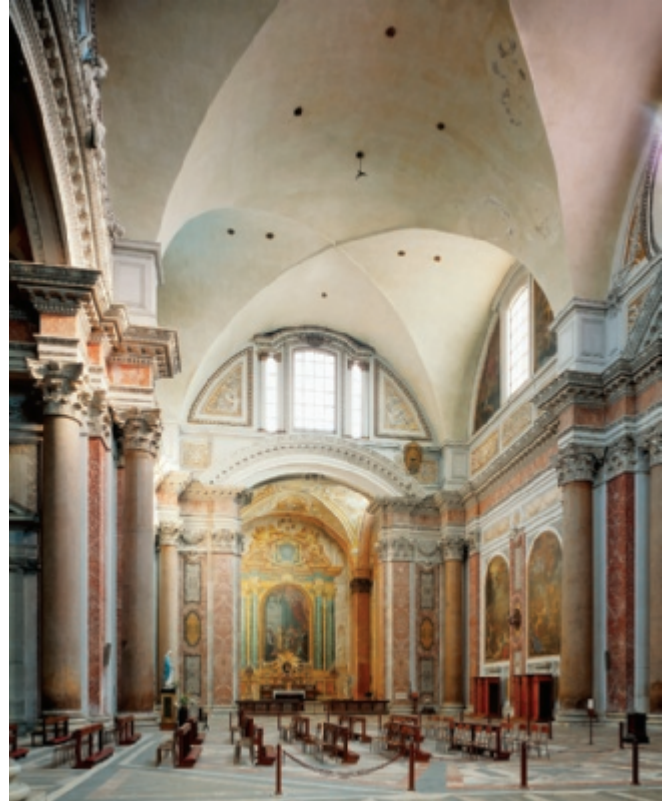
Roman hall with groin vaults (Baths of Diocletian, now Santa Maria degli Angeli, Rome, Italy, ca. 298–306)
