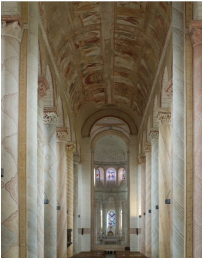
Medieval barrel-vaulted church (Saint-Savin, Saint-Savin-sur-Gartempe, France, ca. 1100)
