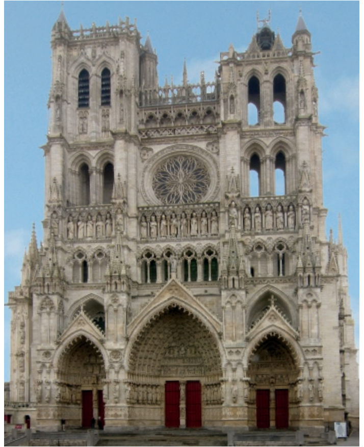
West facade of Amiens Cathedral, Amiens, France, begun 1220
